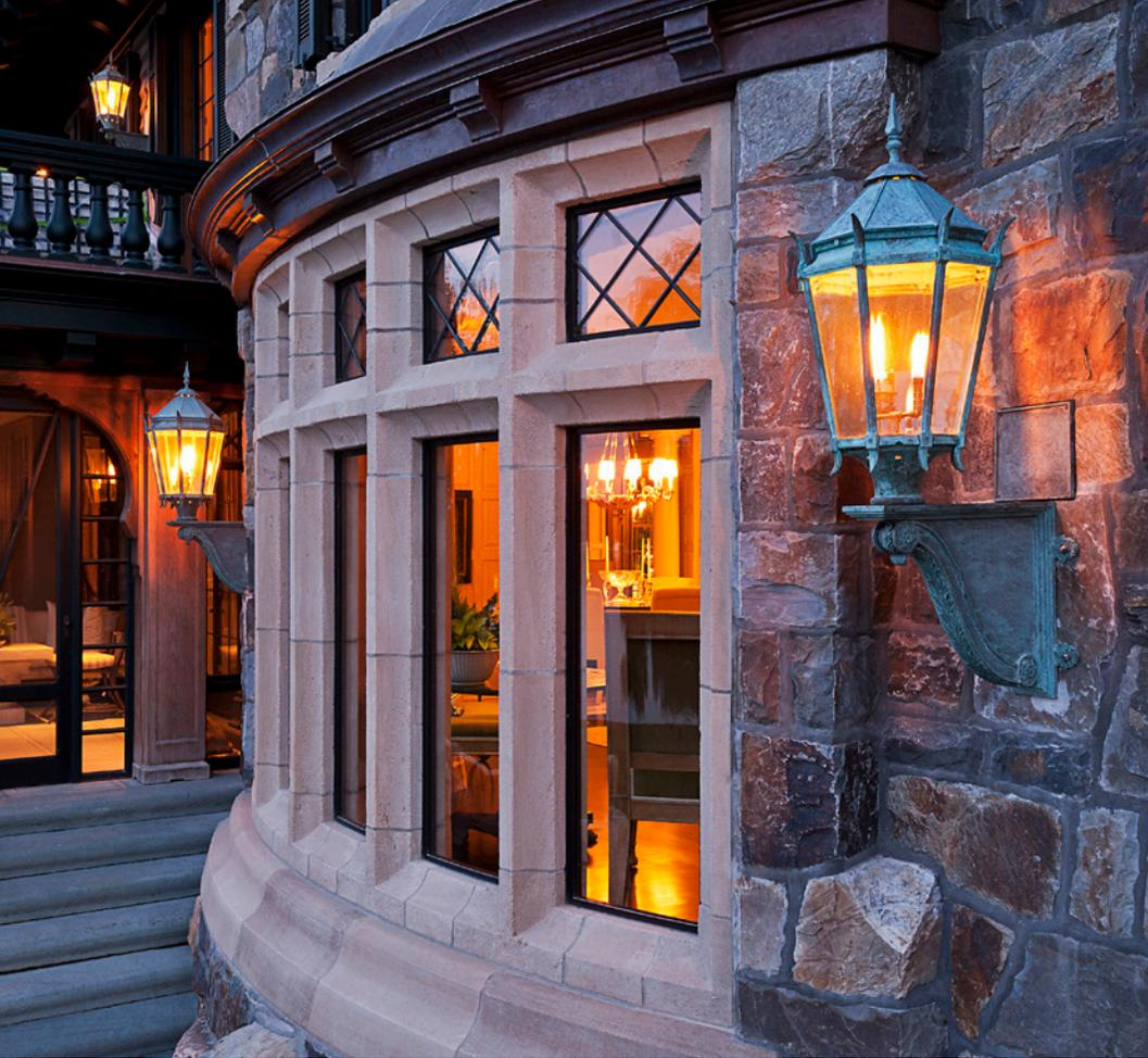
The five fixed curved-on-plan windows are located near the first-floor entry and provide sweeping views of the lake. They were curved to a modest inside radius of 201-3/8" and were glazed with curved-on-plan glass to fit frames measuring 22" by 61".
